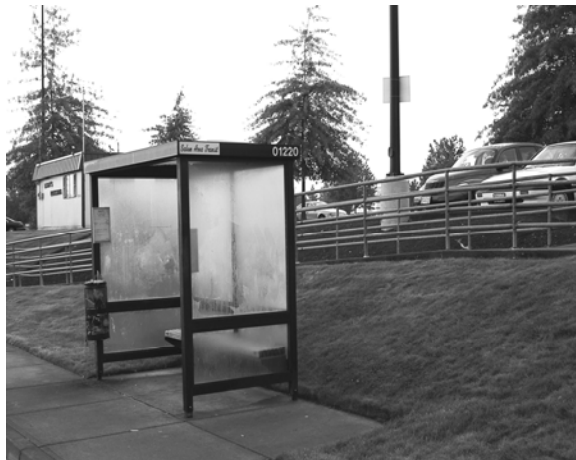
Clean and well-maintained bus stops are important in attracting new riders to the public transit system
